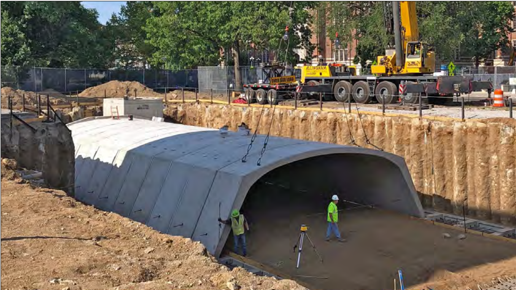
Figure 46. Underground stormwater basin in front of the University of Michigan Museum of Art
