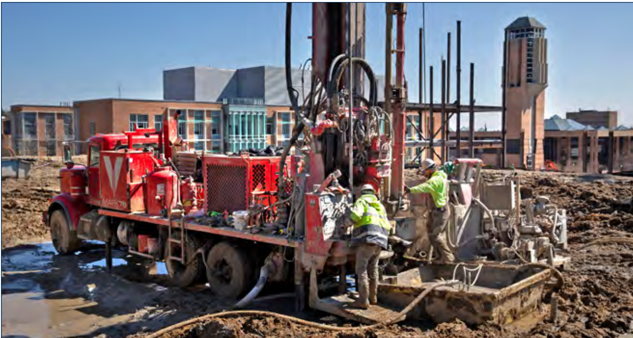
Figure 05. Geothermal drilling on Hayward Street
